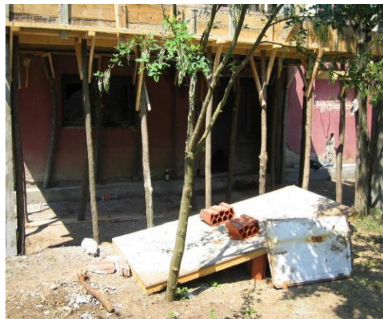
The balcony is being reinforced and concreted
