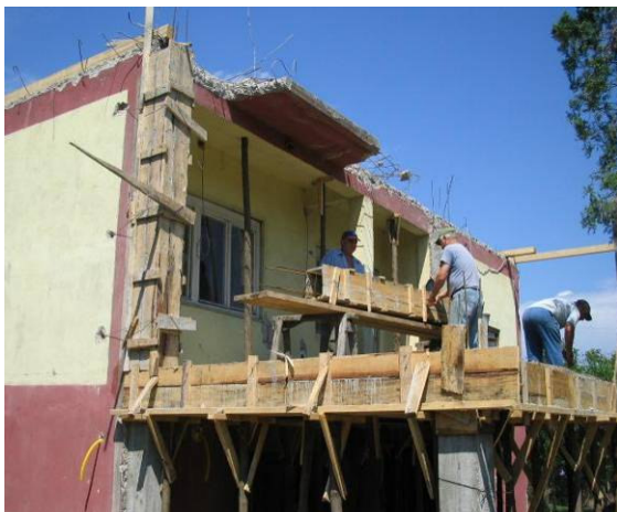
The balcony is being reinforced and concreted
