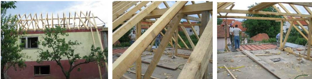
As you can see on the photos the main focus during the last week was to complete the roof. What we have done is that we raised the timbers a bit higher than normal and we got a large space on the attic. It can be used as a place where children can sleep during summer camps.
